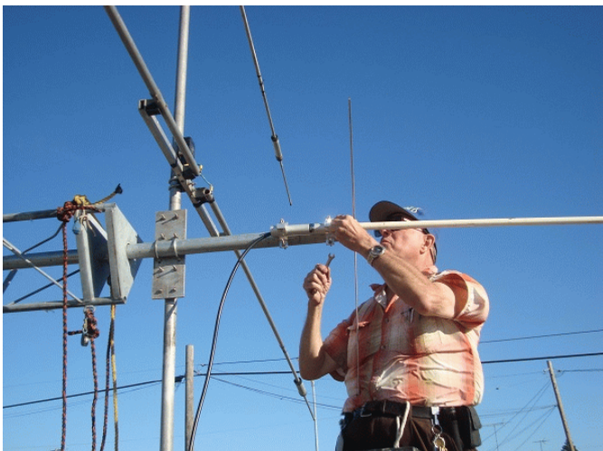
Wally KA6YMD attaching vertical to top of tower
